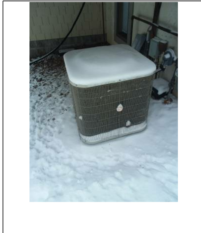
Fins are very dirty and should be cleaned.
