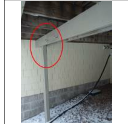
Beam attachment to the post is improper.
