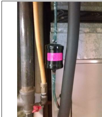
Filter dryer showing some signs of corrosion.
